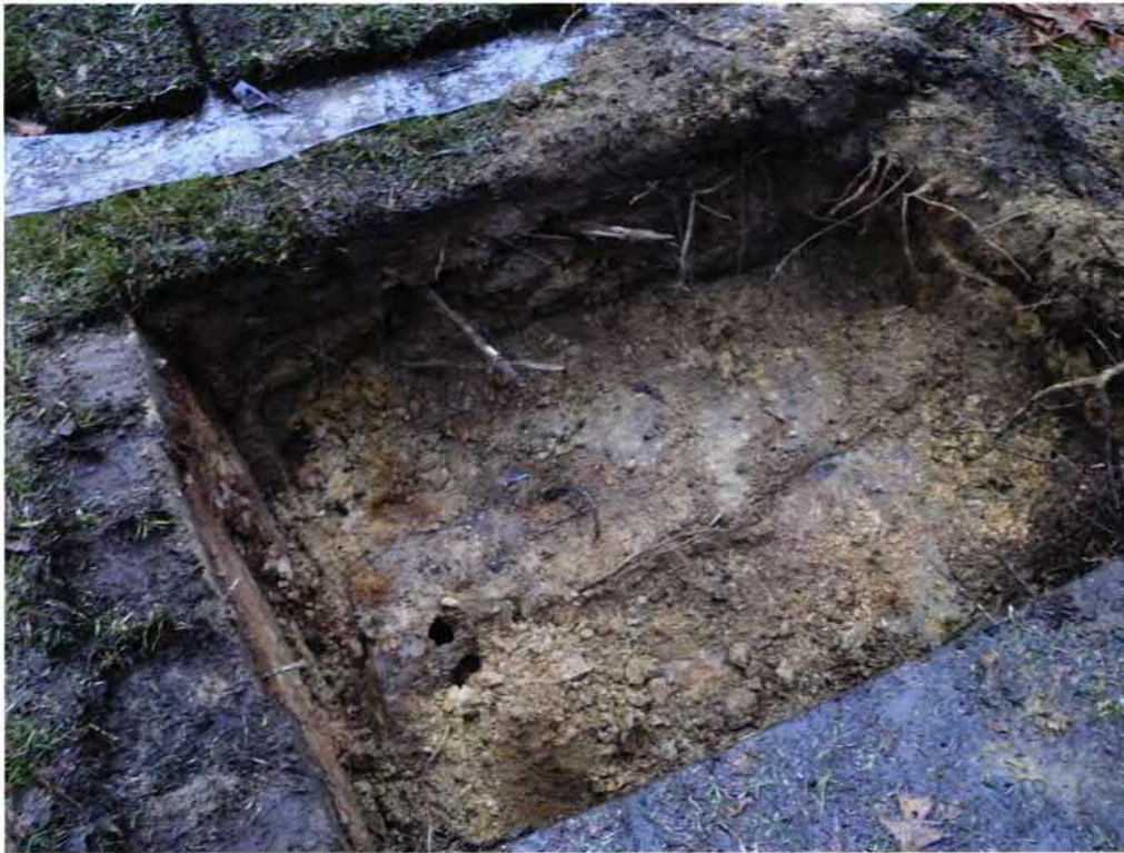
Picture 3: UST 338 Ash-2 excavation in progress.
